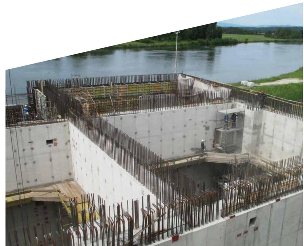
The BB2 building was designed to contain the alternative safety injection system (ASI), the alternative auxiliary feedwater system (AAF) and the BB2 safety power supply. In addition to the BB2, the project includes a well for pumping groundwater for additional supply to the alternative systems for safety injection and power supply for the cooling water system, for the beyond-design basis events.
