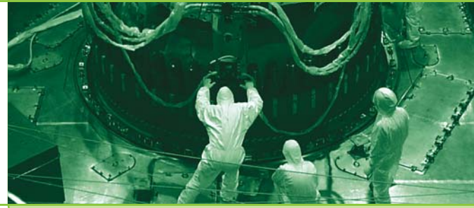
bolt tensioning of the reactor vessel head 4.2*
