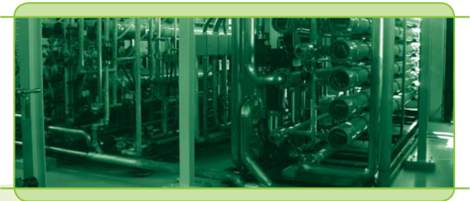
a part of the demineralised water treatment system - reverse osmosis 9.1*
